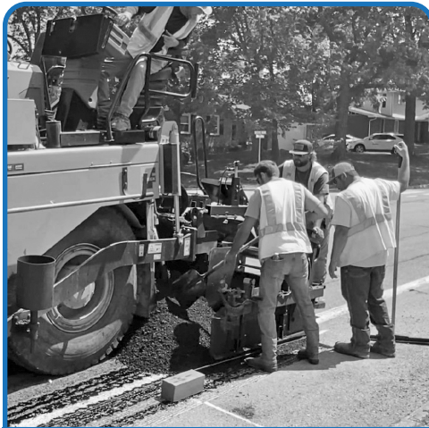
Crews spread asphalt to create a speed hump on Shepard Boulevard.
