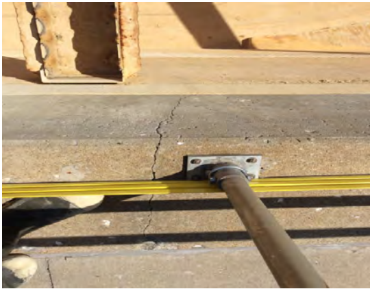
Crack in Top of North Wall in Primary Basin No. 1.
