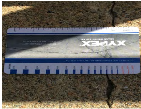
Crack Comparator Measurement at Top of Wall.
