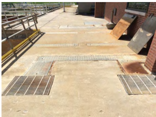
Cracking and Popouts in Top Slab of Tunnel near Primary Basin No. 1.
