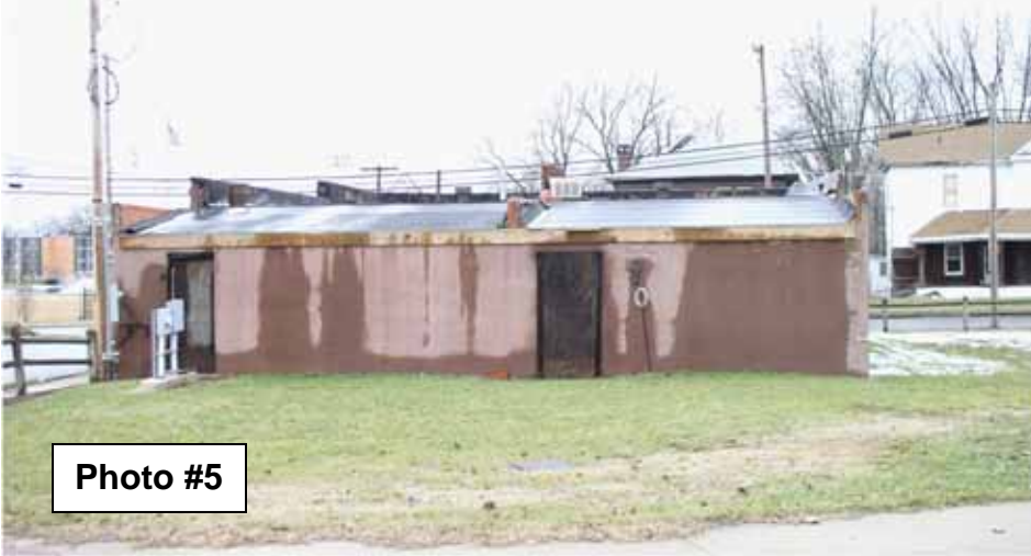
Felt paper not secured in areas of roof. No gutters on fascia board.
