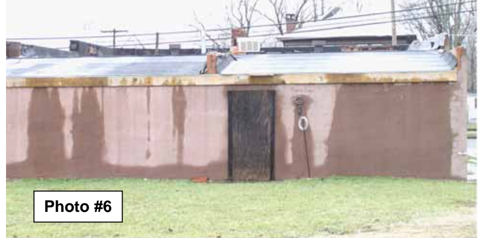
Felt paper rolled onto wooden roof. No gutters on back side.
