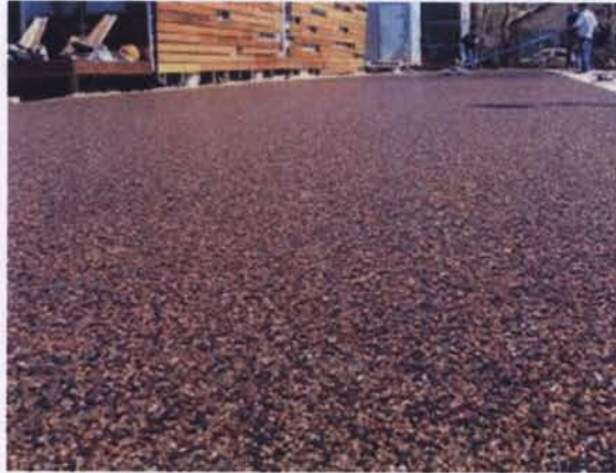
Recycled glass used as a pervious parking lot.
