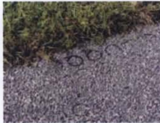
Eroded trails can expose plastic grid below.
