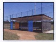
ATKINS DUGOUTS Perspective of typical new dugout construction. Two infield facing entrances are shown in blue and a exterior facing entry way is shown in orange. Dugouts also consist of a sloping roof as appose to a flat roof construction.
