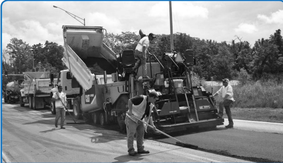
Soon after winter ends, Columbia Public Works uses City staff and private contractors to perform annual street maintenance including asphalt overlay.
