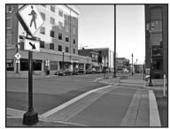
along Eighth Street from Walnut to Cherry. The project included decorative bricks, plantings, ADA—compliant sidewalks, ramps, handrails, landings and crosswalks with flashing beacons. The crosswalk beacons are solar powered which not only reduces energy costs but also eliminates the need to connect them to the electric grid.
