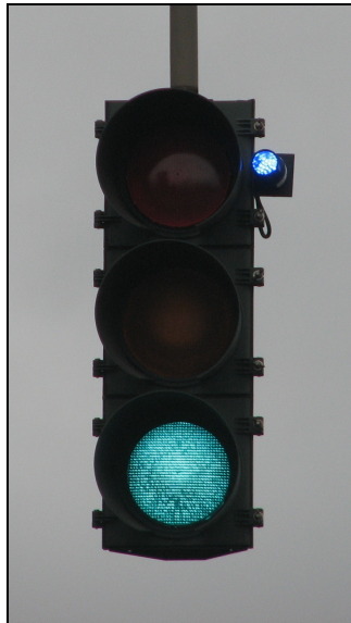
FIGURE 3 A Close-up of a Traffic Signal with a Blue Light Feedback Device at the NE Tillamook Street Site
