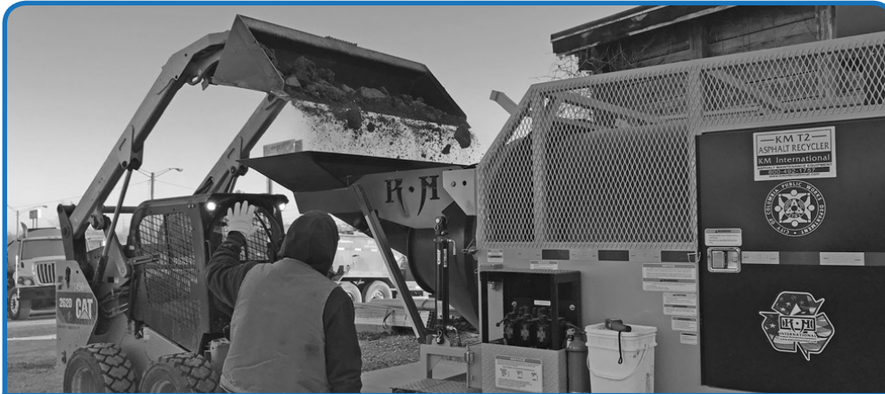
The City purchased an Asphalt Recycler in 2018 for making an asphalt hot mix to repair potholes throughout the year.
