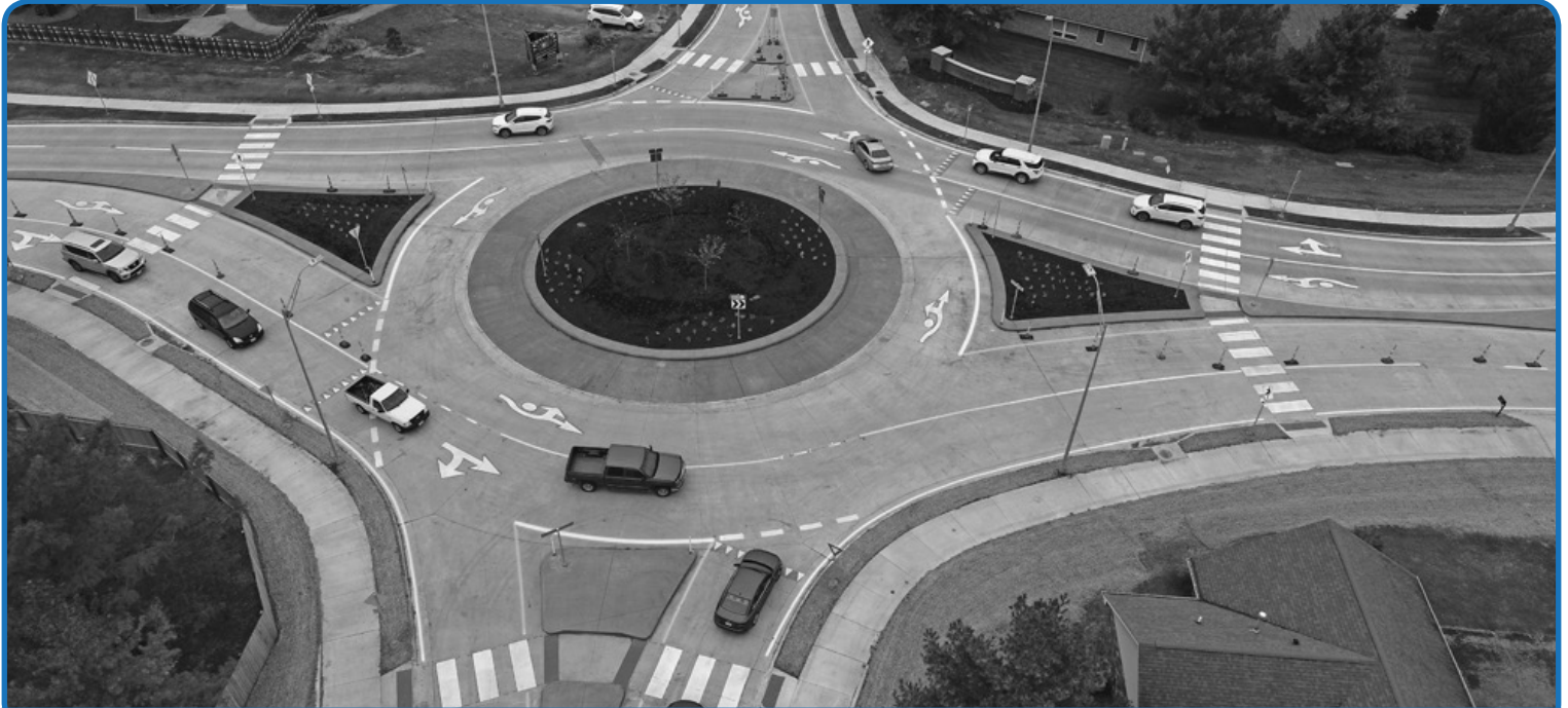
The Green Meadows Road and Forum Boulevard roundabout includes street lighting, sidewalks, crosswalks and pedestrian safety islands.
