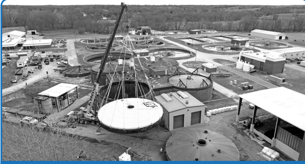
The improvements to the digester complex will allow for a more efficient and effective mixing of wastewater sludge. Photo credit: River City Construction, LLC
