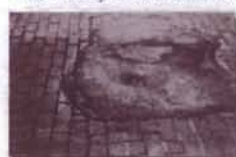
Area filled in with asphalt (photo by Jill Downs)
