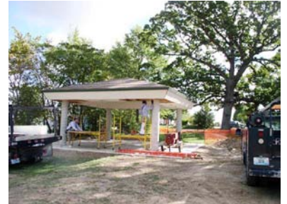
Louisville Shelter Construction
