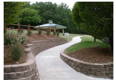
MLK Shelter and Retaining Walls
