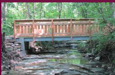
Wilson Bridge Replacement
