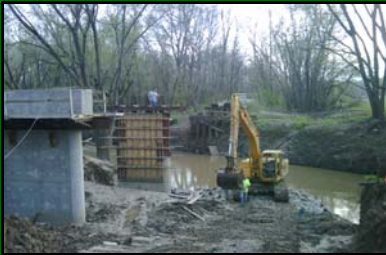
MKT Bridge #12 Construction
