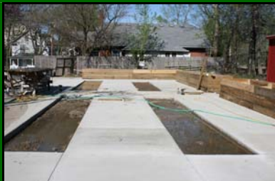
Paquin Garden Area Concrete
