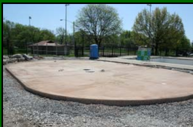
Douglass Sprayground Pad
