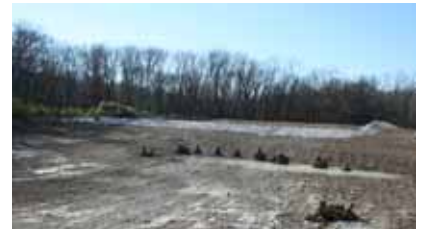
Nifong Lake Dam Work
