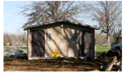
New Restroom at LOW
