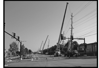
Lacing the 80-foot-tall transmission and distribution poles on Fairview.
