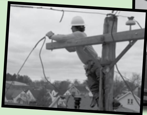
Lineworker Andrew Smith replaces electric lines in Ohio.
