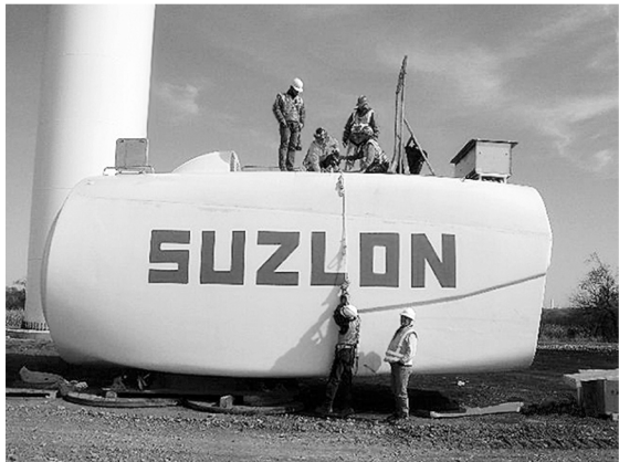
left: Workers prepare to hoist the nacelle of turbine #27, one of Columbia's designated turbines. below: Representatives from Columbia Water & Light, Associated Electric, and Wind Capital Group join Mayor Darwin Hindman and City Manager Bill Watkins at the signing ceremony.
