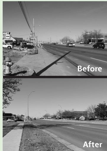
The recent electric undergrounding project near Garth Avenue on the Business Loop.
