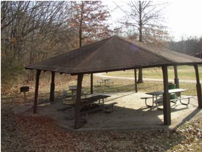
GNA Shelter Removed
