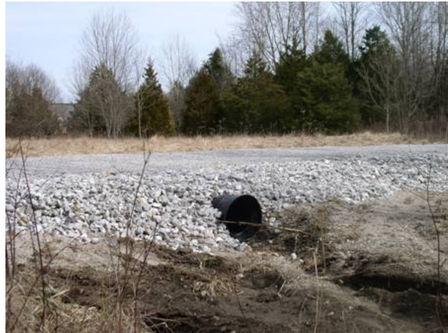
Culvert replacement on Bear Creek Trail
