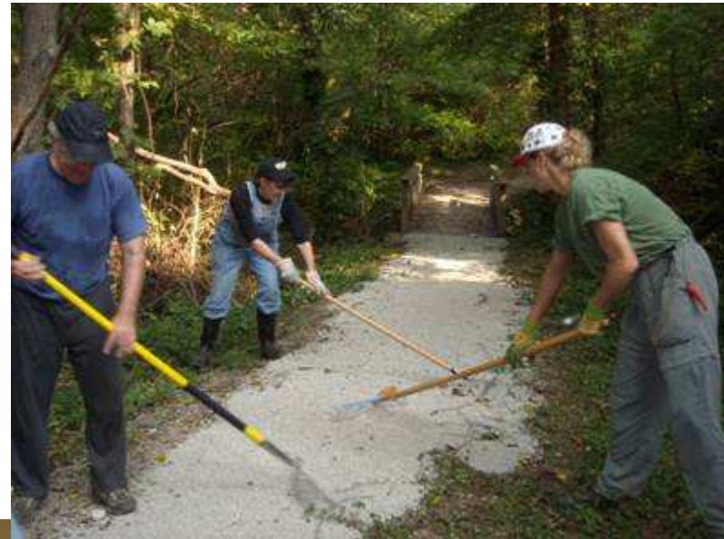
Trail Resurfaced with New Rock
