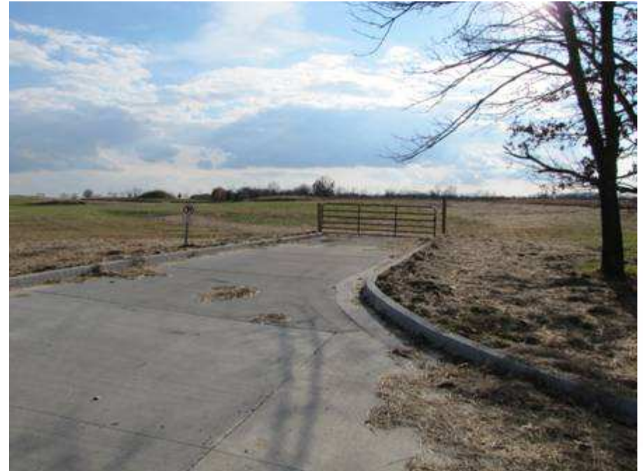
Extended trailer back-up ramp
