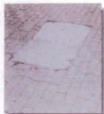
Utility cut repaired with concrete (photo by Jill Downs)
