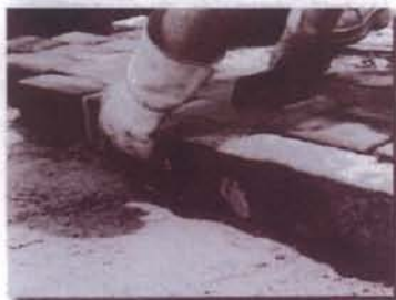
Note that bricks are placed with raised name on the side (photo by Jason Swisher)
