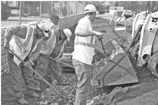
A Public Works Stormwater Operations crew spreads rock in a new bioswale on Ashley Street.
