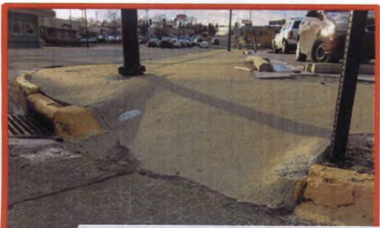
Fourth & Broadway • No detectable warning • No contrasting color • Slope too steep • Not aligned with crosswalks (either direction)
