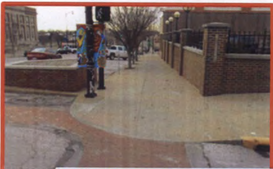
Seventh & Broadway • No detectable warning • No contrasting color • Slope too steep
