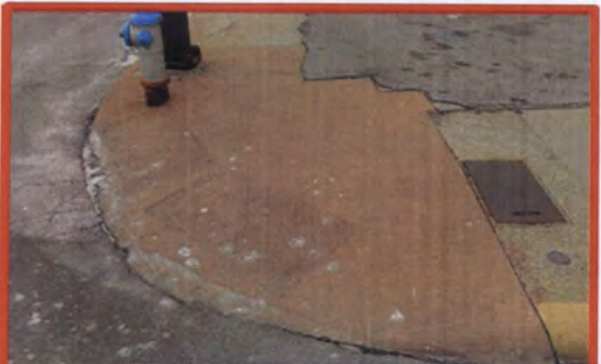
Fifth & Broadway • Detectable warning stamped in concrete • Slope too steep
